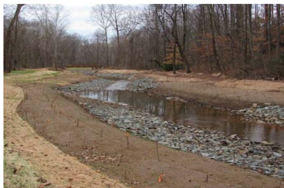
Photo 4. Example 2 - Stream banks after reshaping and armoring. Source: The Nature Conservancy & City of Charlottesville
