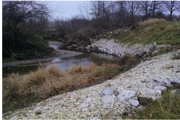
Photo 2. Example 1 - Jordan Creek after bank shaping with rock toe protection. Source: LT Leon Associates
