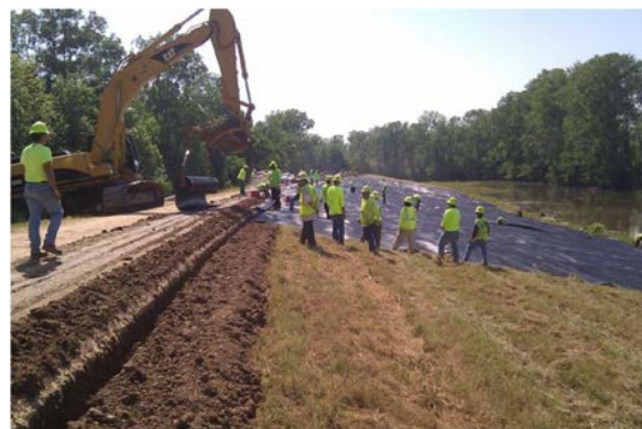
Photo 20. Levee maintenance. Source: USACE
