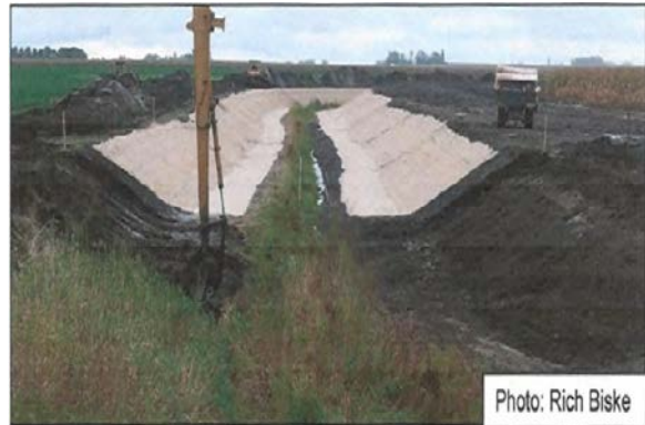
Photo 26. Example 2 - Two-stage channel during final restoration. Source: The Nature Conservancy
