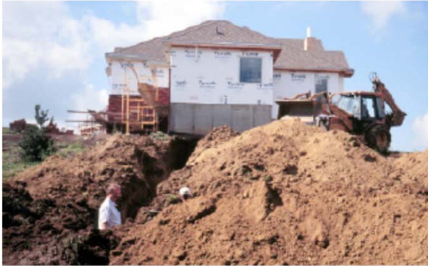
Soils are often disturbed during construction.
