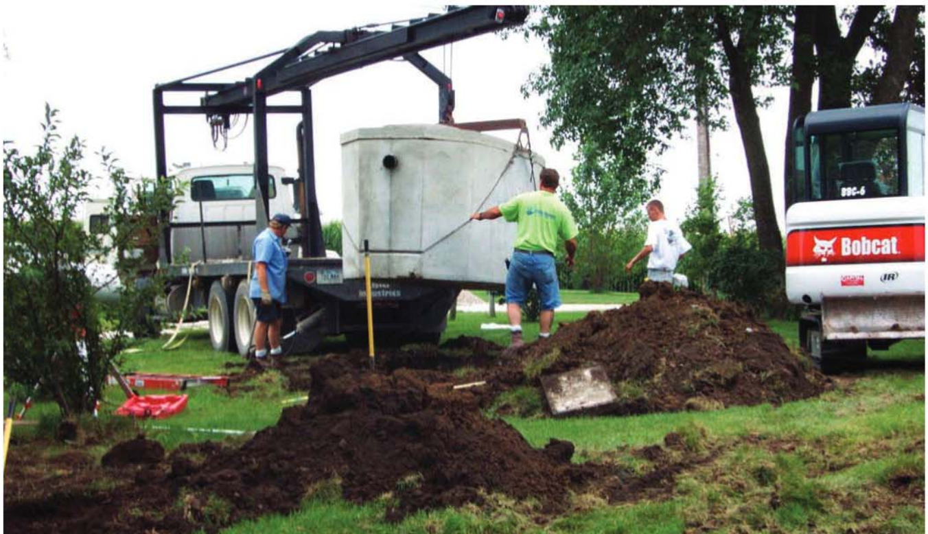
Installation of a new septic system.
